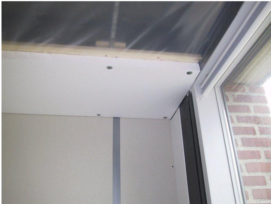
Figure 2.22. Mounting the insulation foam plates at the ceiling of the test rooms.
