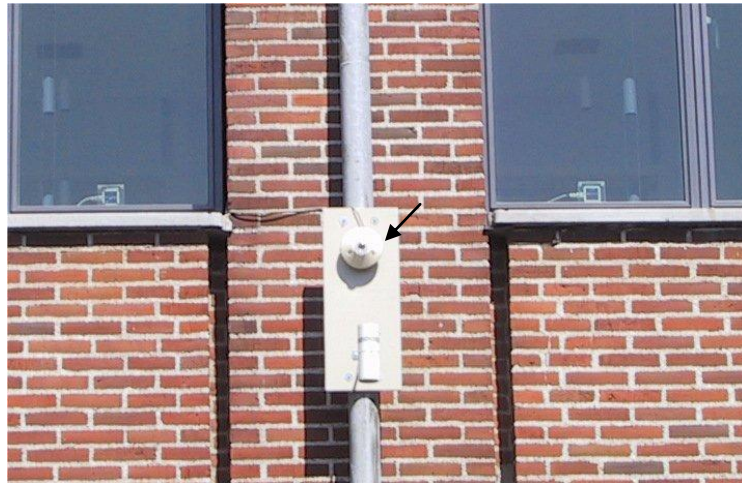
Figure 3.13. The vertical external pyranometer.
