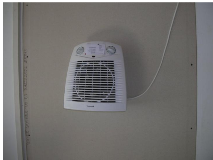
Figure 3.21. Electrical heater for conditioning of the room next to test room B.
