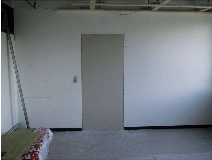
Figure 2.12. The doorway in the shared wall in test room B after closing.
