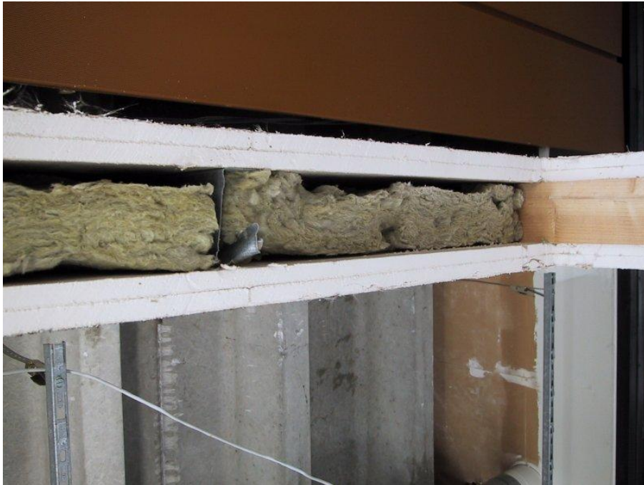
Figure 2.11. The construction of the shared wall in room B – top of the doorway before closing.
