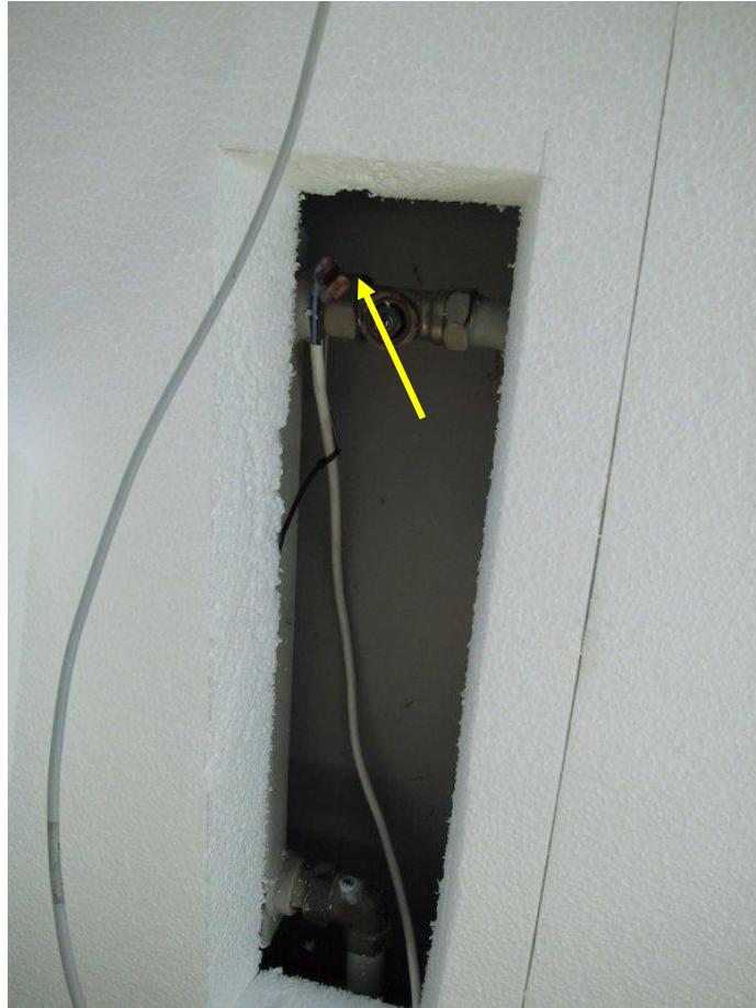
Figure 3.11. Temperature sensor for the alarm.
