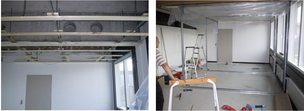
Figure 2.21. The wooden boards and plastic foil forming the top of the ceiling in the test rooms.
