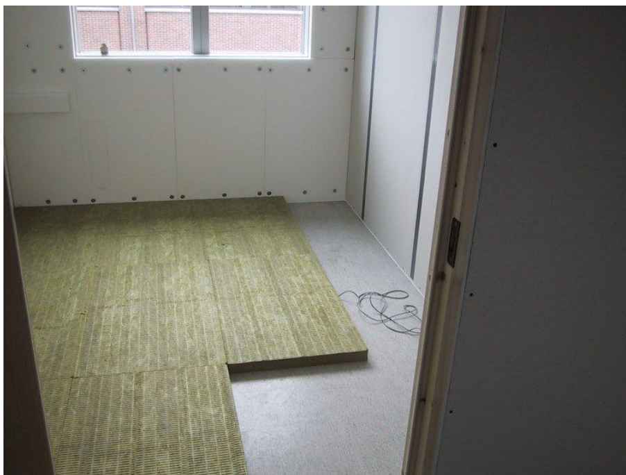
Figure 2.23. Insulation of the floor of the test rooms.
