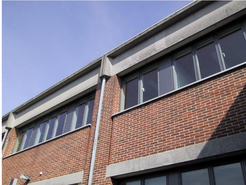
Figure 2.5. The column in the façade between the two test rooms.
