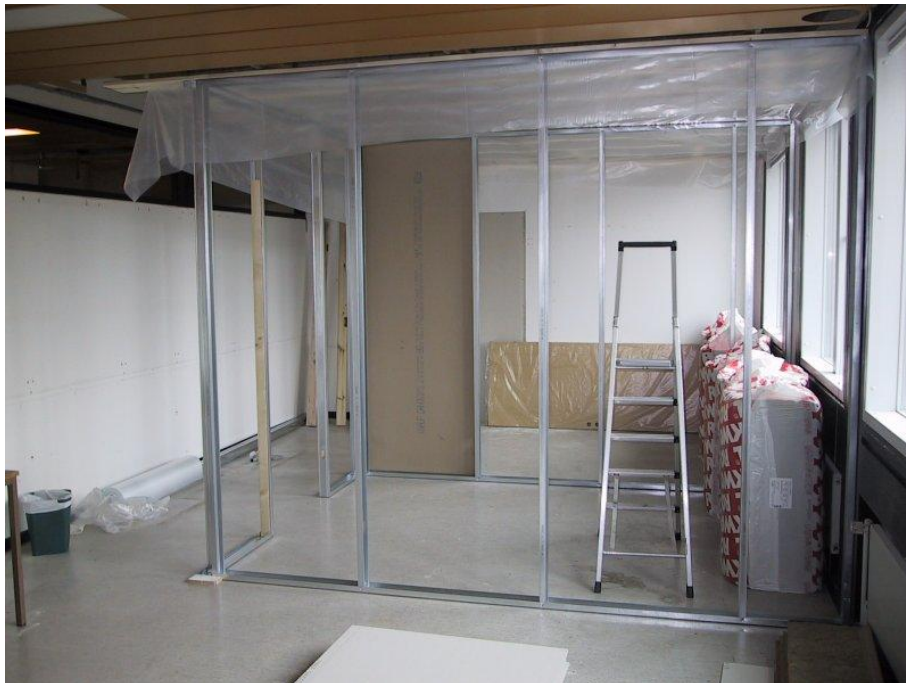
Figure 2.7. The steel skeleton of the two test rooms.
