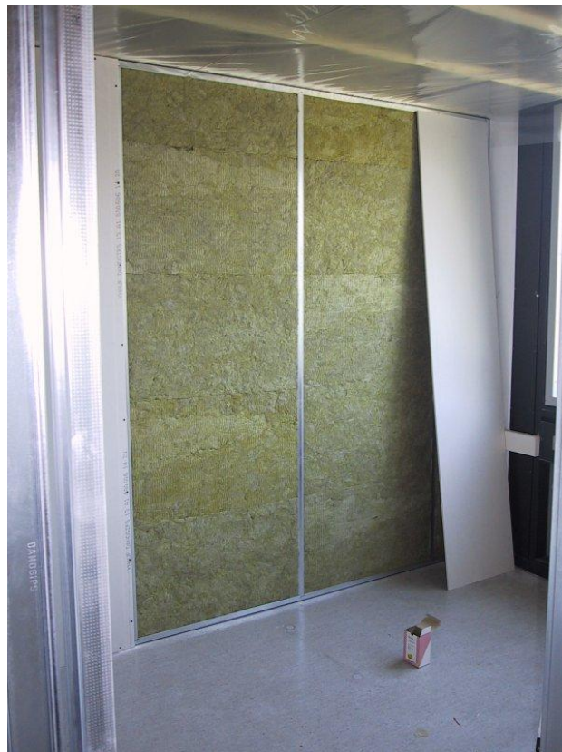
Figure 2.9. One wall after insulation and the gypsum plates being mounted.
