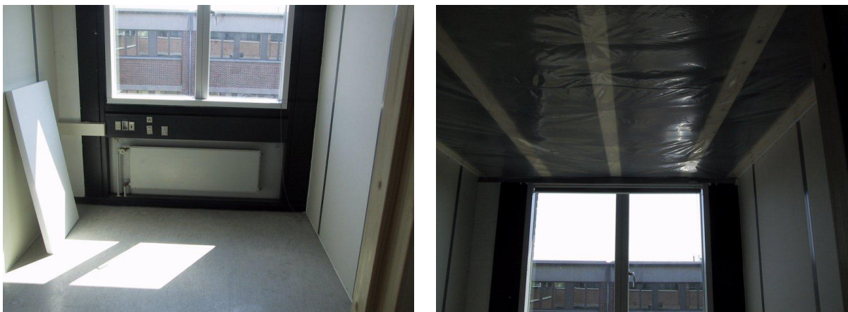
Figure 2.18. Pictures of the inside of the original external wall.
