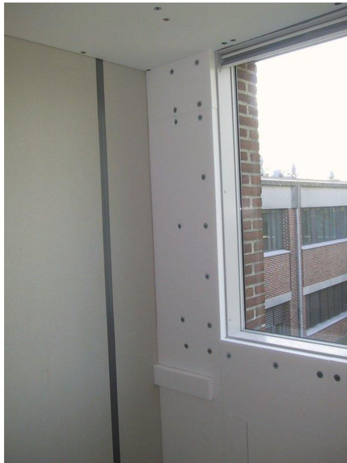
Figure 2.20. Close up of the insulation foam at the window frame.
