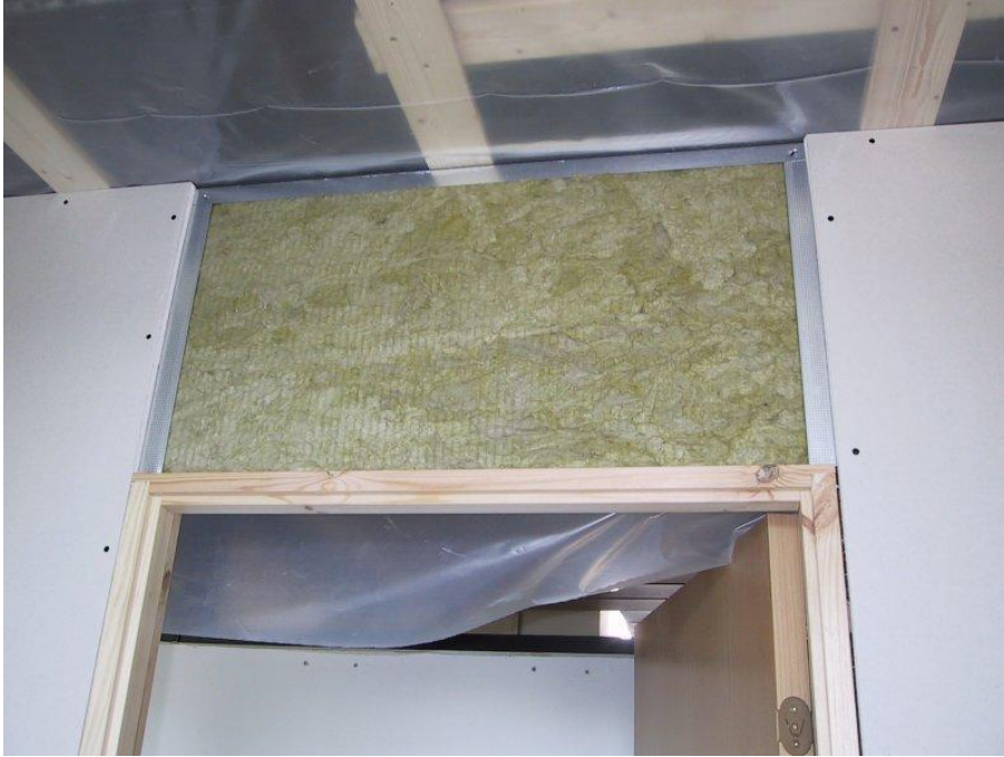
Figure 2.10. Sectional bars mounted at each side of the field above the entrance doors of the test rooms.
