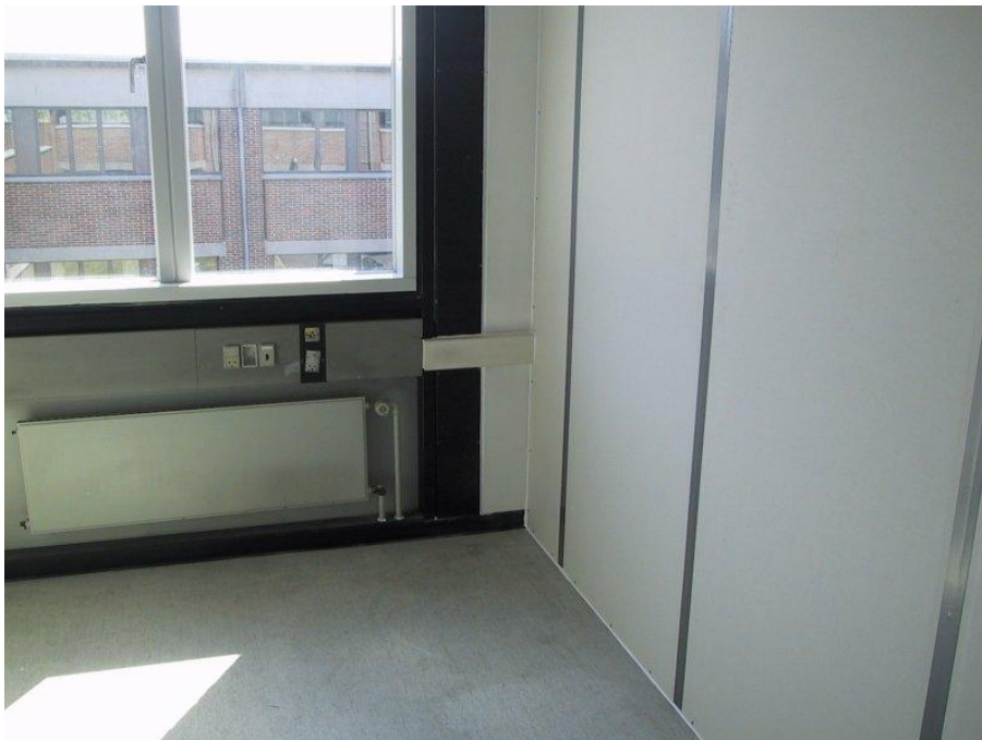
Figure 2.13. Sealing of joints and corners.
