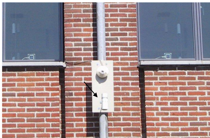
Figure 3.7. Shielded ambient temperature sensor on the column between the two test rooms. Shielded by two concentric cylinders as the air temperature sensors in the test room.
