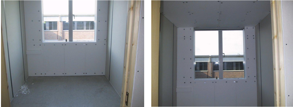
Figure 2.19. Pictures of the inside of the facades after insulation with insulation foam plates.
