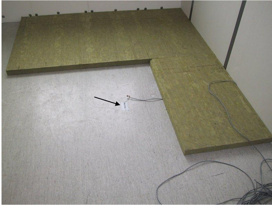
Figure 3.6. Temperature sensor mounted on the floor before the installation of the insulation on top of the existing floor.
