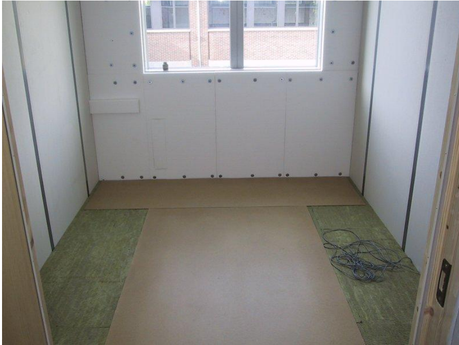
Figure 2.24. A hard fibre boards are located on the top of the floor insulation.
