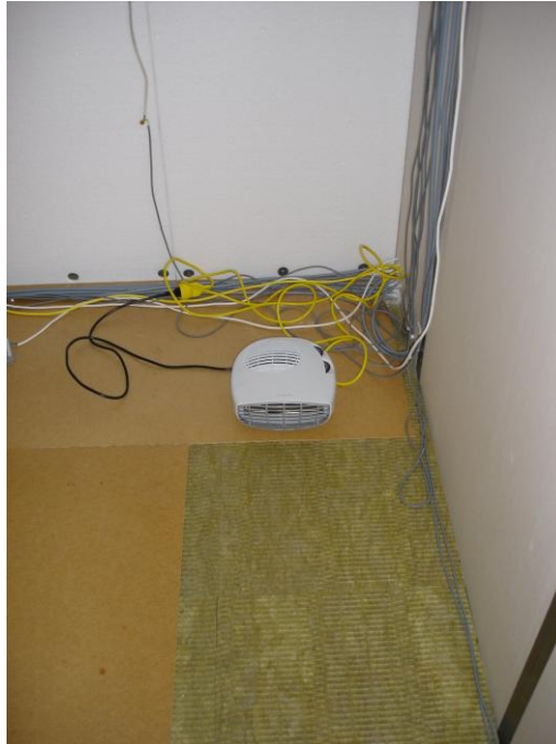
Figure 3.18. One of the electrical heaters of the test rooms.
