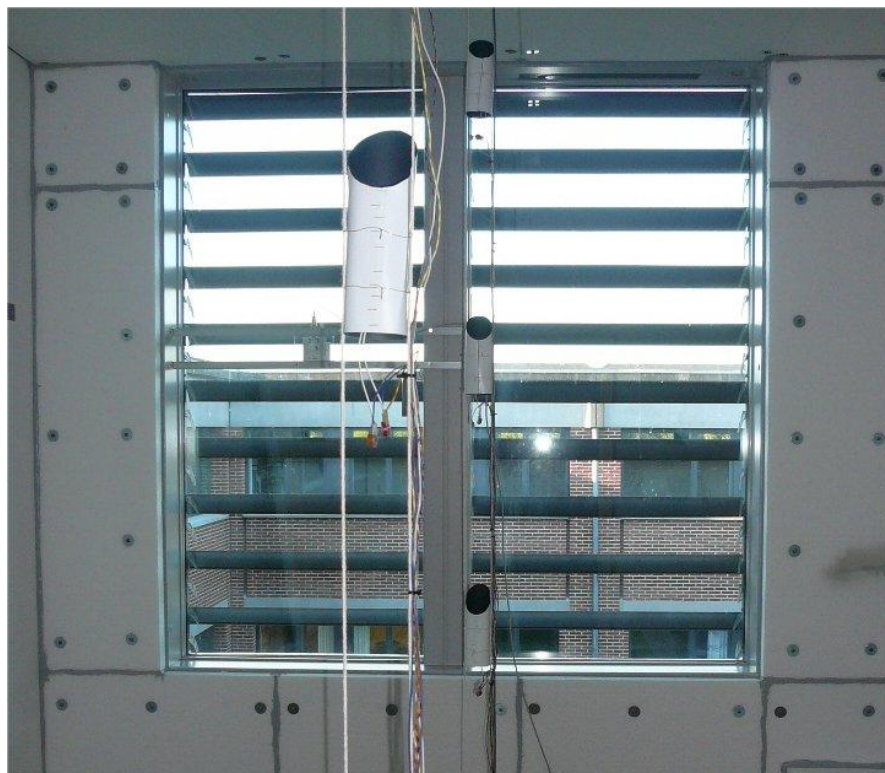
Figure 2.3. The Faber solar screening system with only half the number of lamellas.
