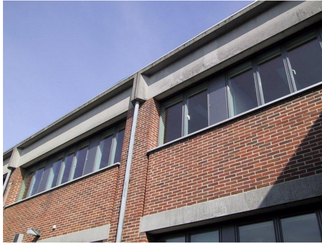
Figure 1.5. The column in the façade between the two test rooms.
