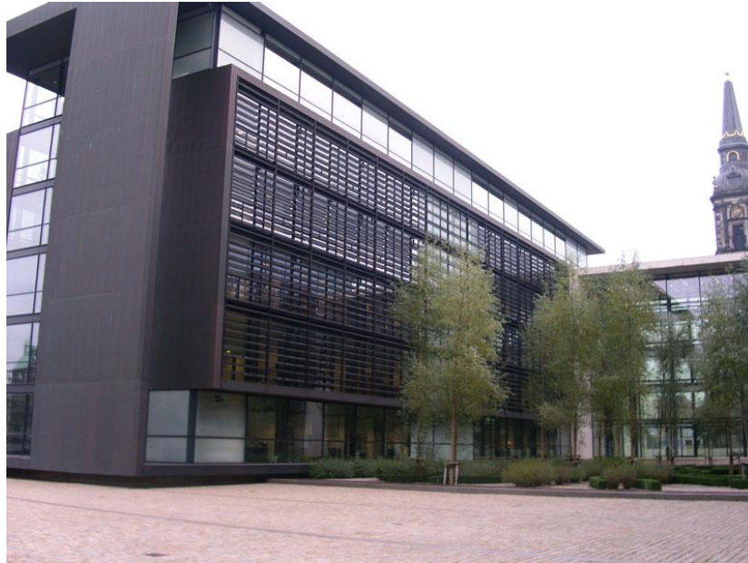
Figure 6.2. One south façade of the Nordea building.
