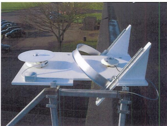
Figure 5 The solar measuring station.
