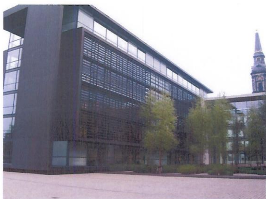
Figure 22 One south façade of the building.
