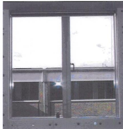
Figure 2 The view out of a traditional low-e window with solar control coating in test room B. g-value of the window: 0.37.
