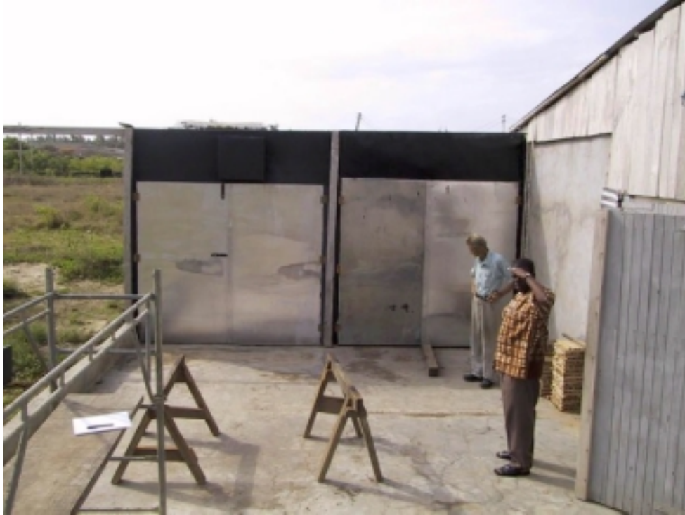
Figure 9. Both solar kilns after conversion of the forced open air dryer into a kiln.
