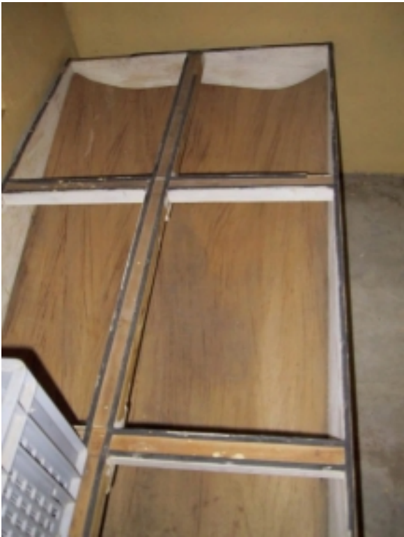
Figure 7. Floor in a pressure chamber made of plywood.
