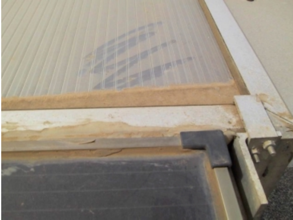
Figure 7. The photo clearly shows the dust deposit on the solar air collector and PV-panel.
