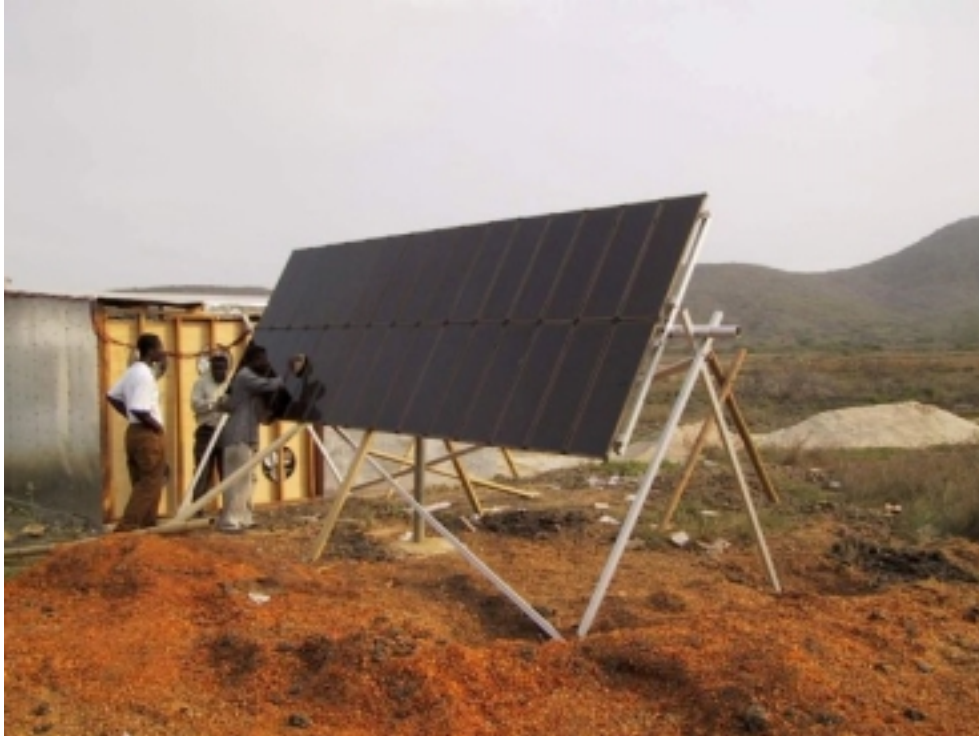
Figure 3. The PV-panel of the forced open air dryer – here turned to face west – being cleaned
