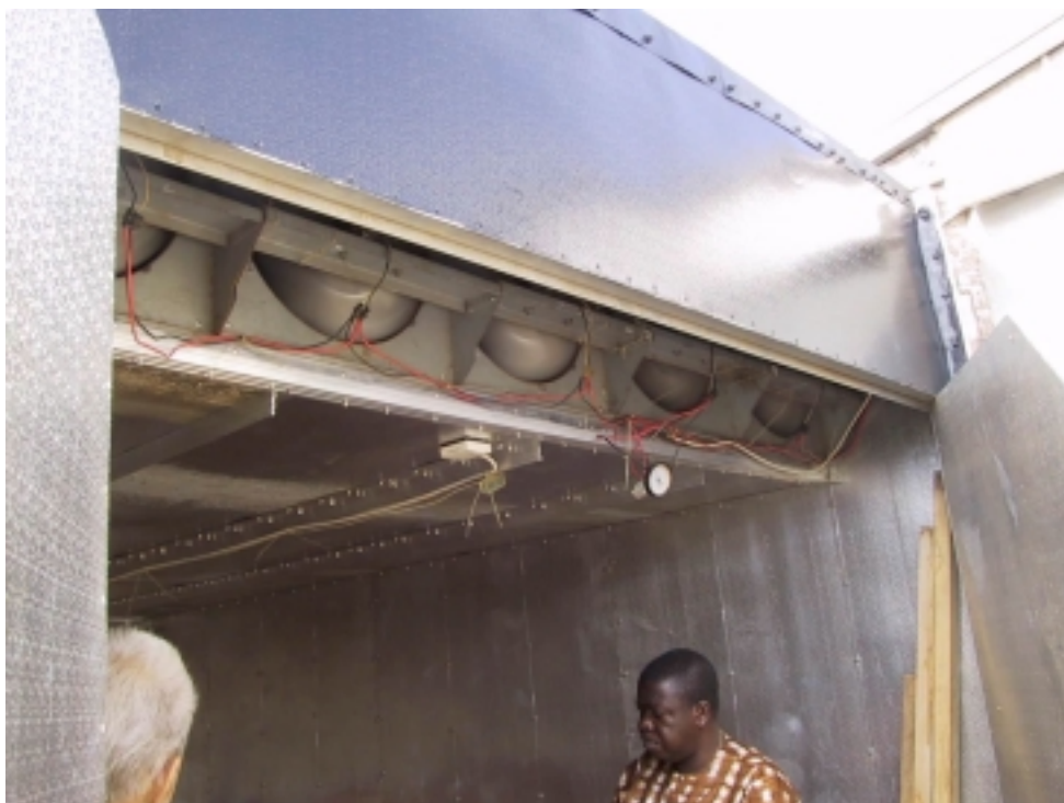
Figure 8. The daytime fans of the new solar kiln after conversion from a forced open air dryer.
