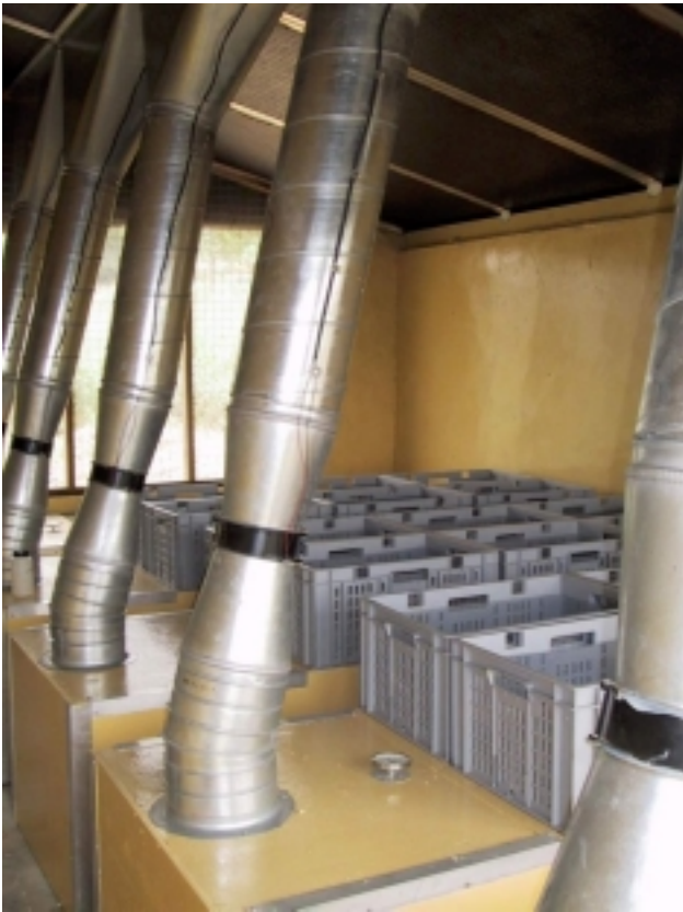
Figure 3. The five drying units inside the building containing the solar crop dryer.
