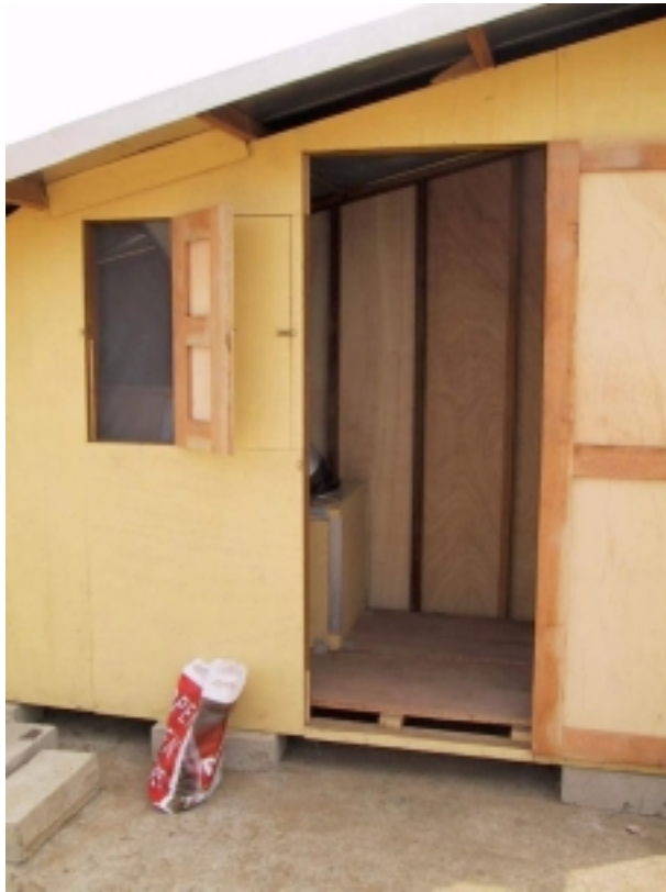
Figure 2. The solar fish dryer seen from the east. The dryer has two hatches in the east wall with insect net and an entrance door.
