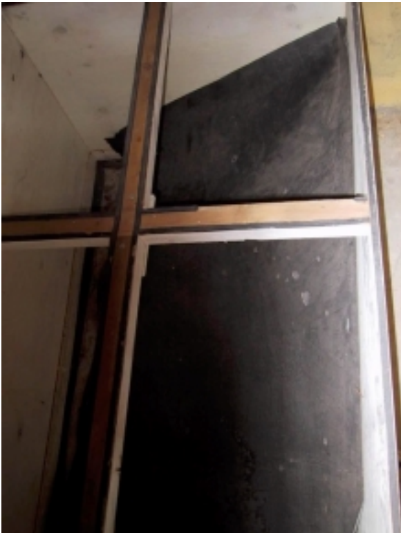
Figure 8. Floor in a pressure chamber made of sheets of 5 mm insulation foam.
