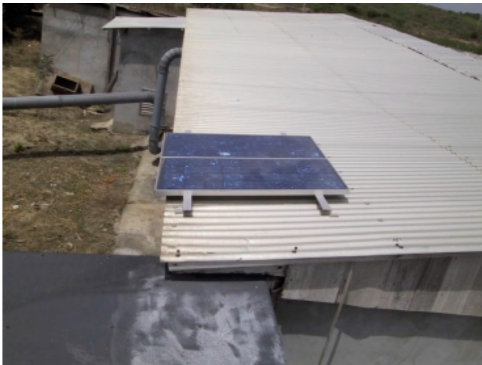
Figure 10. Two PV-panels for changing the batteries powering the night fans.
