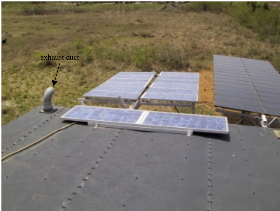
Figure 7. The array of PV-panels for the two solar dryers. For the solar kiln to the left including two panels on the roof of the kiln. The exhaust duct of the kiln is also shown.
