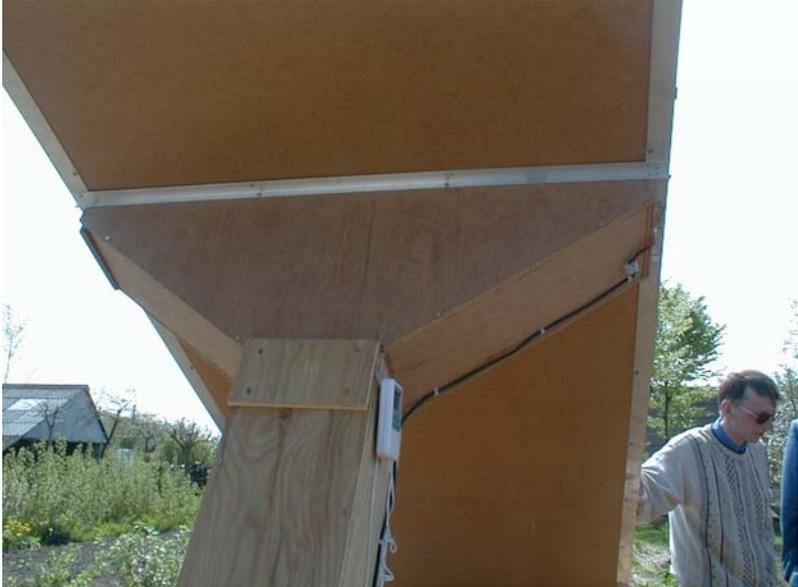
Figure 2.10. The manifold connecting the collector with the duct leading to the fan.
