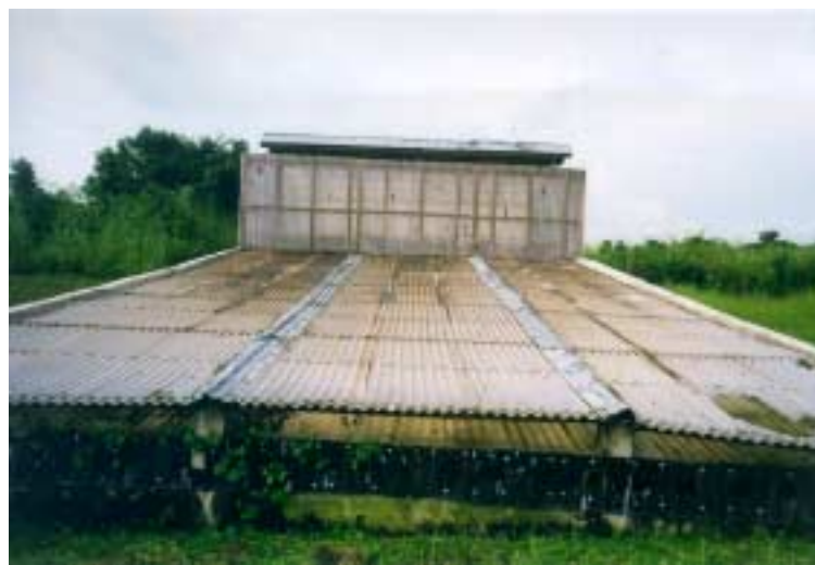
Figure 5.1. One of the solar dryers in Agona Asafo. The top photo shows the drying chamber while the bottom photo shows one of the collectors.
