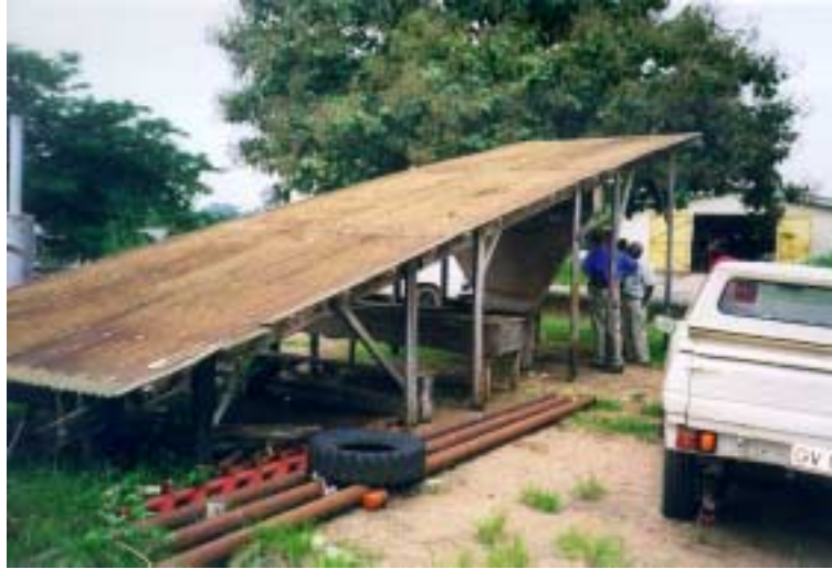
Figure 5.3. Old solar air collector at the Department of Agricultural Engineering.
