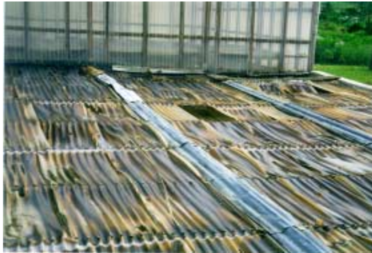
Figure 5.2. Deterioration of the cover of one of the collectors in Agona Asafo.
