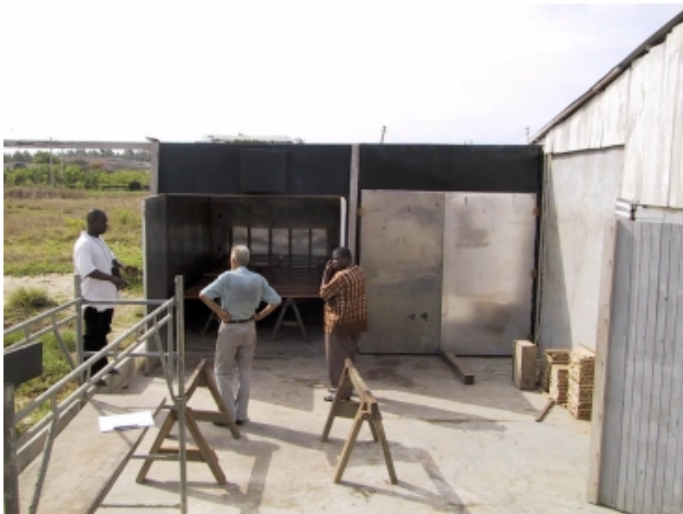
Figure 6.5. The two chambers for the open-air wood dryer (to the right) and the solar kiln (to the left) seen from the north.
