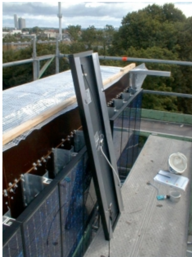
Figure 1.28. Top of the PV-area of one of the solar ventilation chimneys during mounting.
