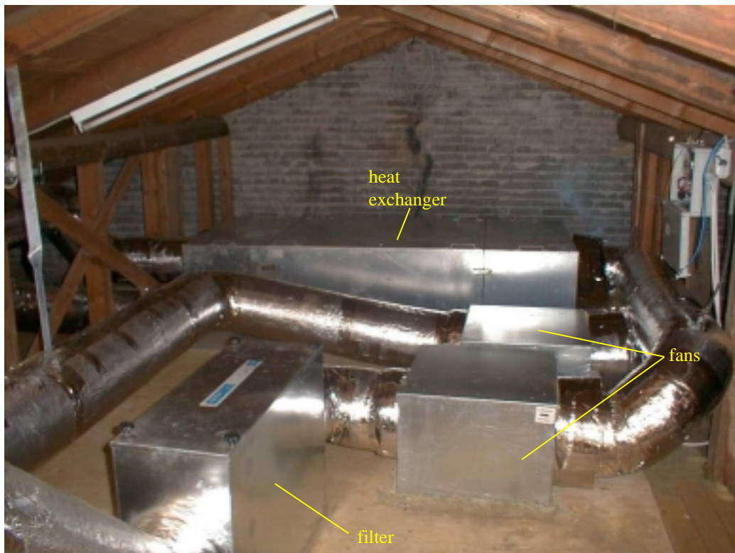
Figure 1.23. The common ventilation system for the C apartments in no. 40 and all the apartments in no. 38.
