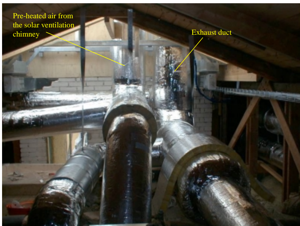
Figure 1.30. Ductworks in the attic to and from one solar ventilation chimney.
