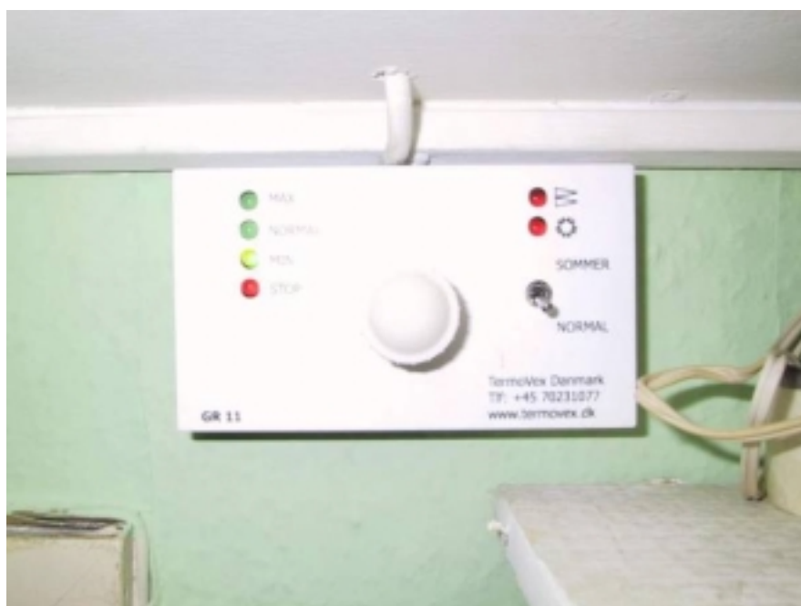
Figure 1.34. The control panel from which the occupants of the A apartments in no 40 may control their ventilation systems.
