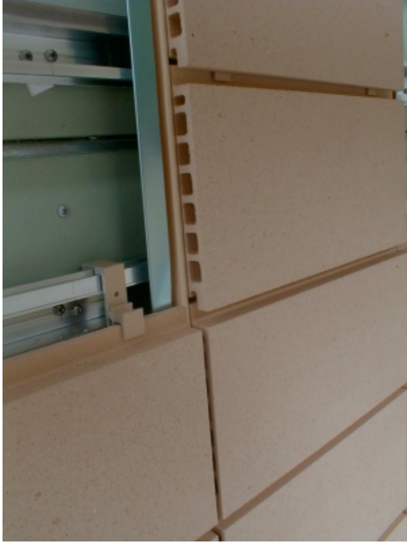
Figure 1.35. The external cladding of the externally insulated facades.
