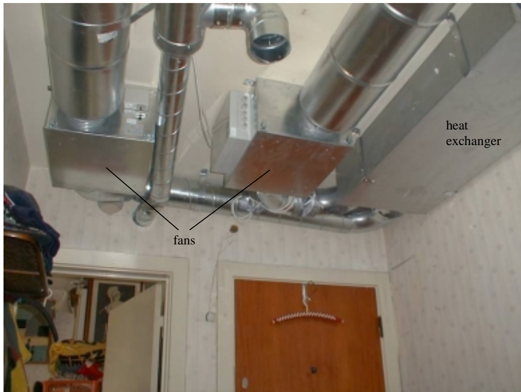
Figure 1.21. The fans and heat exchanger in the hall of the A apartments.
