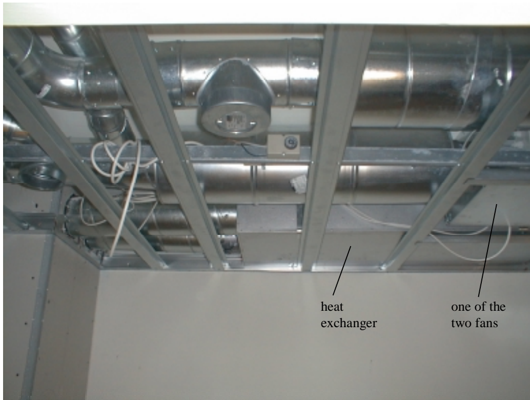
Figure 1.22. The ventilation systems in the B apartments in no. 40.
