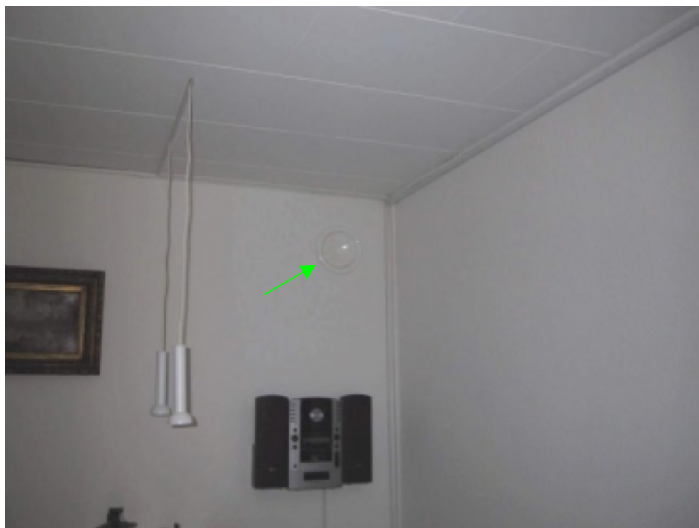
Figure 1.13. Inlet diffuser for letting pre-heated air in from the air gap behind the PV-panels in the south gable.
