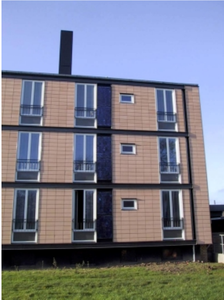
Figure 1.18. The three PV-arrays (one for each floor) at the east facade are connected to the ventilation systems in the A apartments in no. 40.
