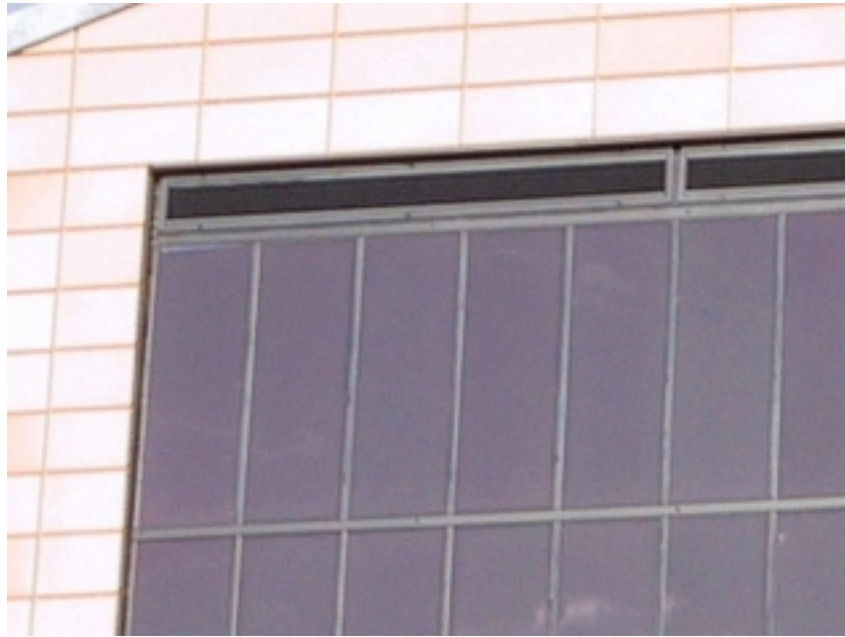
Figure 1.15. Orbesen damper for summer ventilation of the air gap in the PV-gable.
