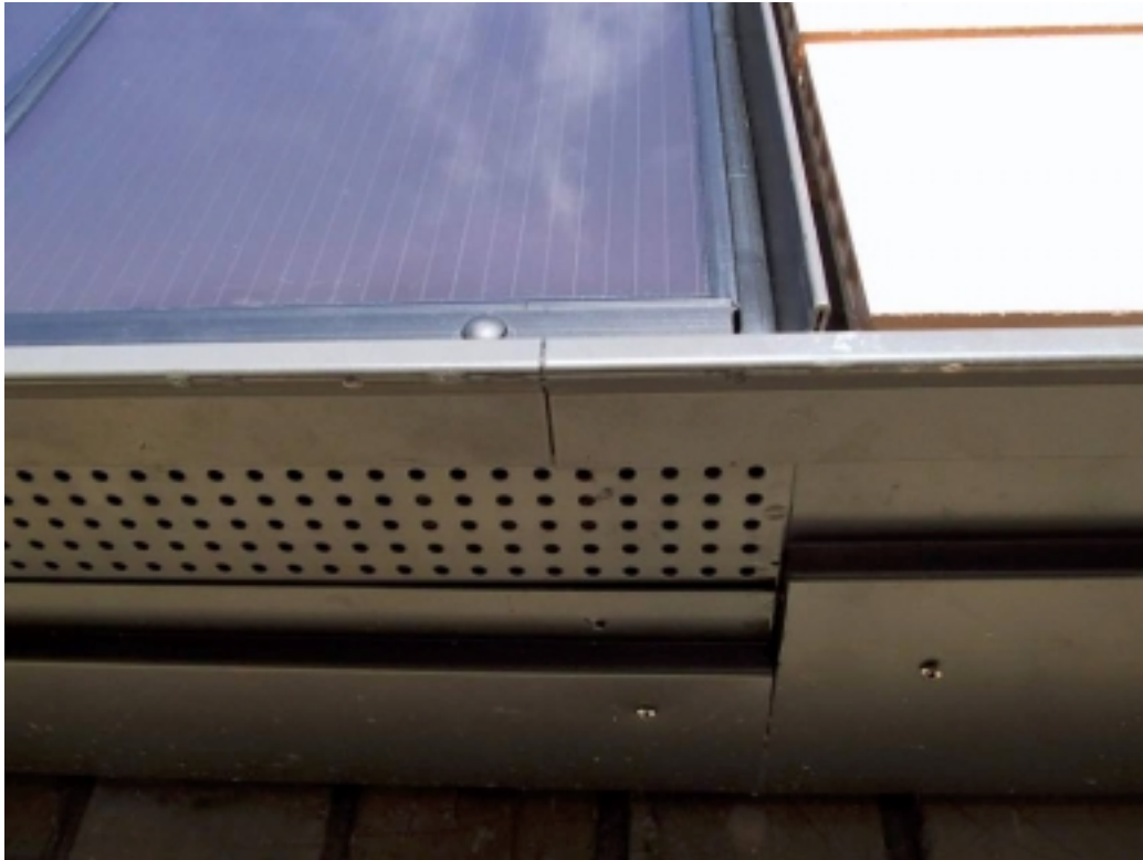
Figure 1.14. The inlet at the bottom of the PV-gable.
