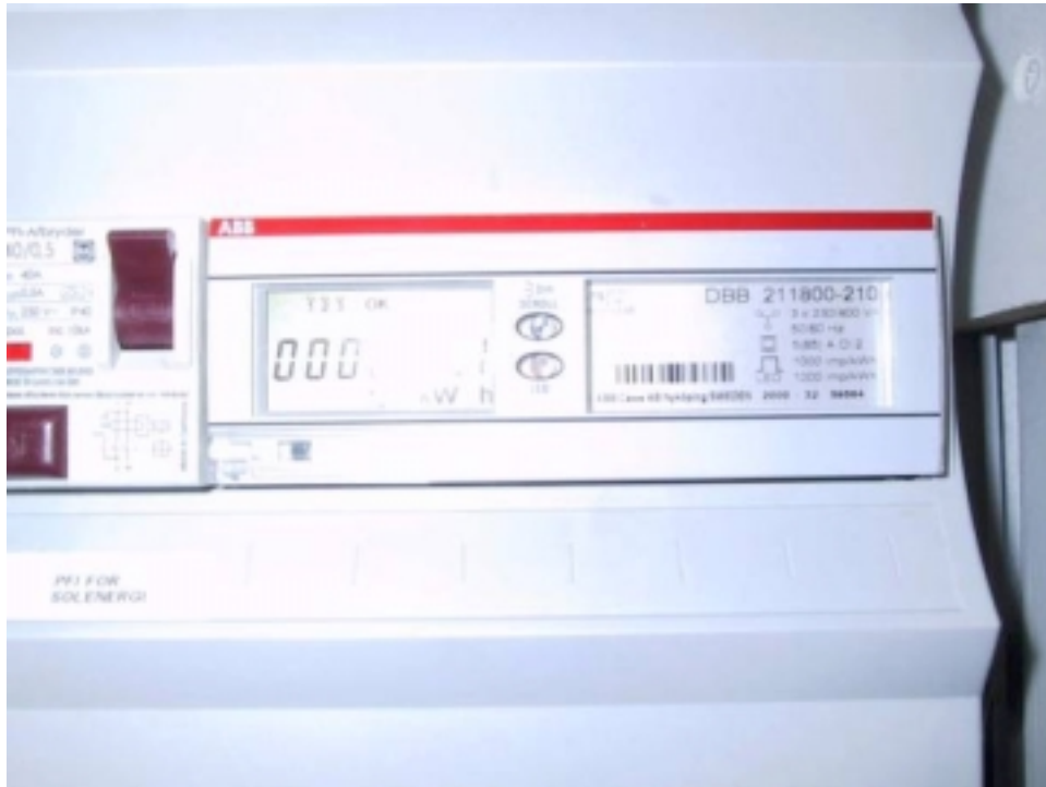
Figure 2.6. The power meter for measuring the energy production of one of the three arrays of PV-panels on the to the 2 nd floor.
