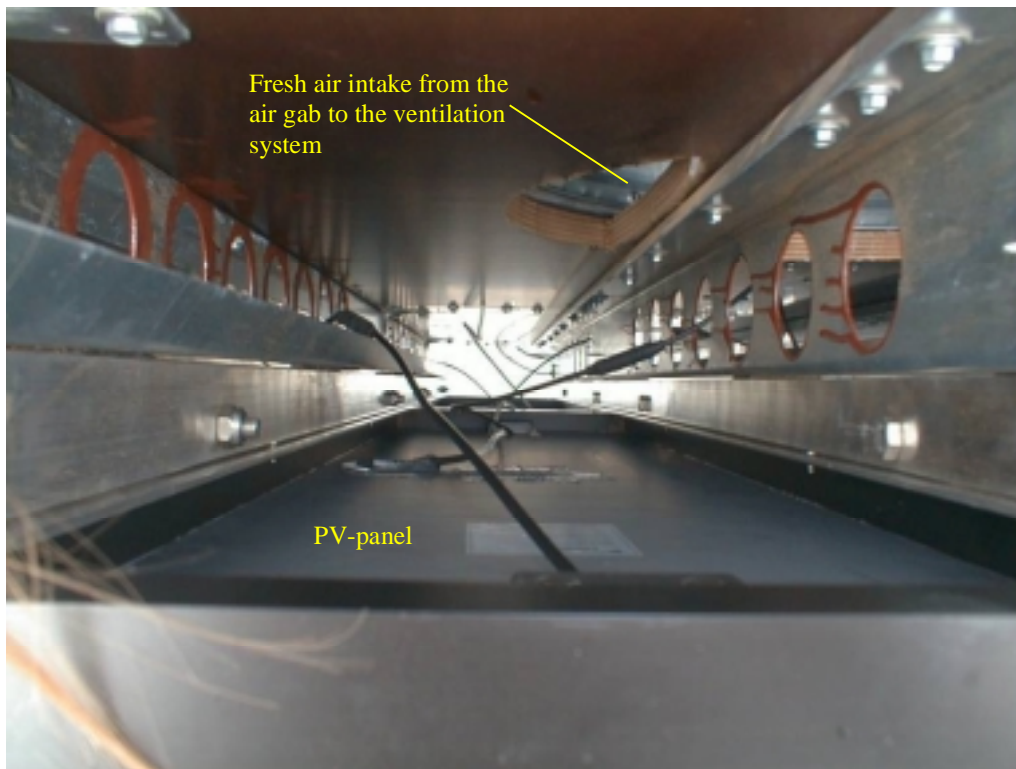
Figure 1.29. View down the air gap behind the PV-panels of the solar ventilation chimneys.
