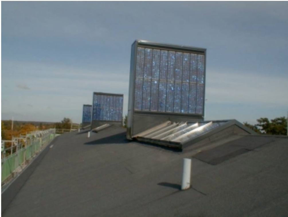
Figure 1.24. Three solar ventilation chimneys on the roof.
