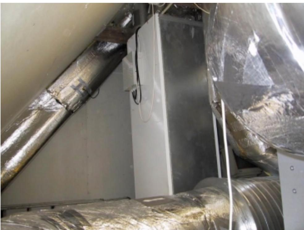
Figure 2.17. The small heat exchanger from AirVex for the top apartments to the left.
