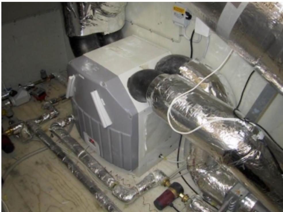
Figure 2.16. The small heat exchanger from Exhausto for the top apartments to the right.
