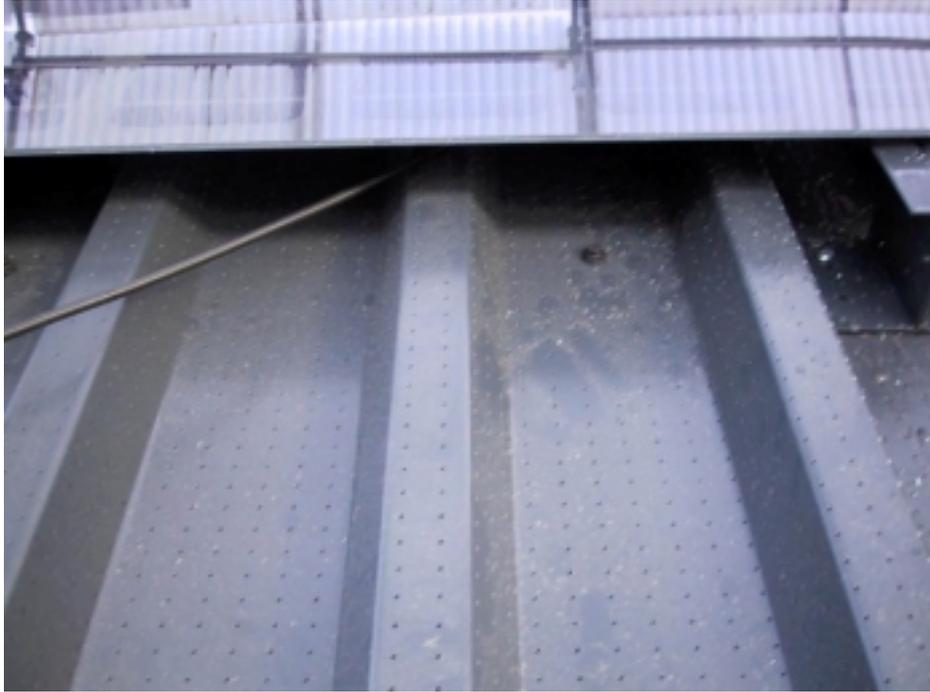
Figure 2.6. The PV-panels mounted on top of the Solarwall sheets.
