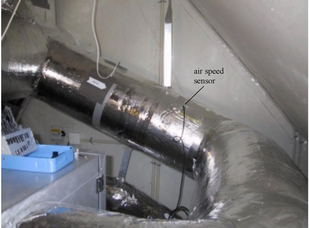
Figure 3.6. Top picture: the inlet duct of fresh air to the large heat exchanger before insulation. Bottom picture: the location of the air speed sensor.
