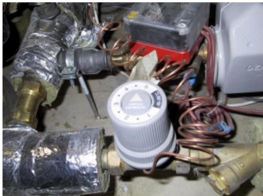
Figure 2.20. Thermostat for controlling one of the heaters in the ventilation systems.
