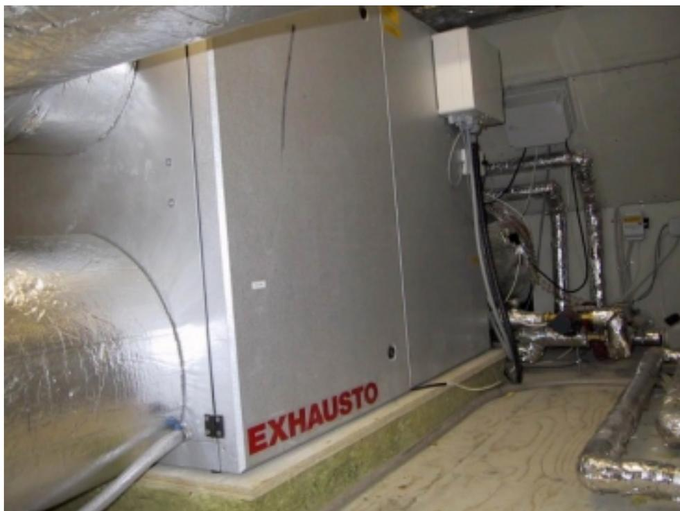
Figure 2.15. The large heat exchanger from Exhausto for 10 apartments.
