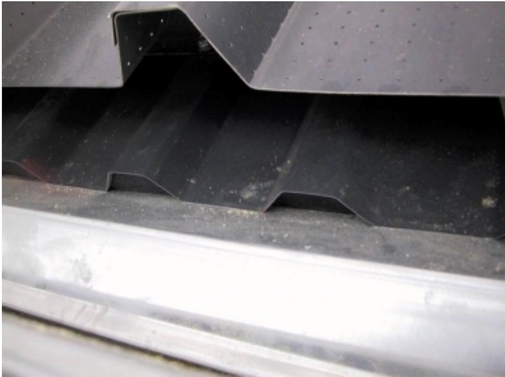
Figure 2.4. The under roofing and the Solarwall sheet.
