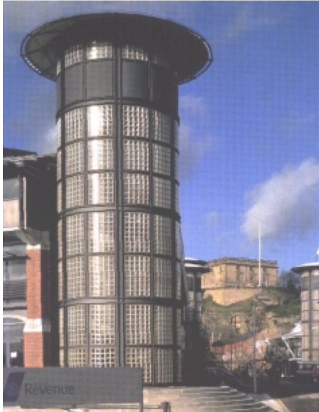
Figur 4.16. The inland Revenue Building (Herzog, 1996)
