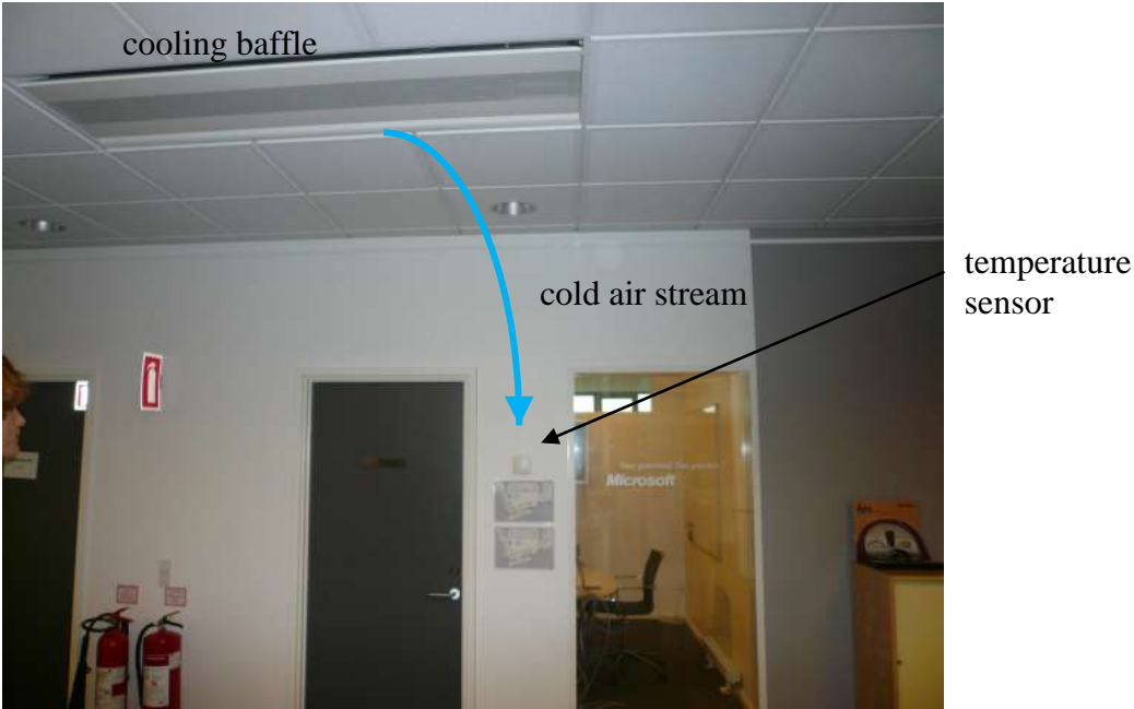
Figure 5.4. Cold air hitting the temperature sensor directly.
