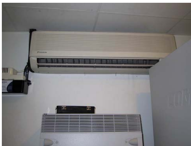
Figur 2. Serverrummets fordampere.
