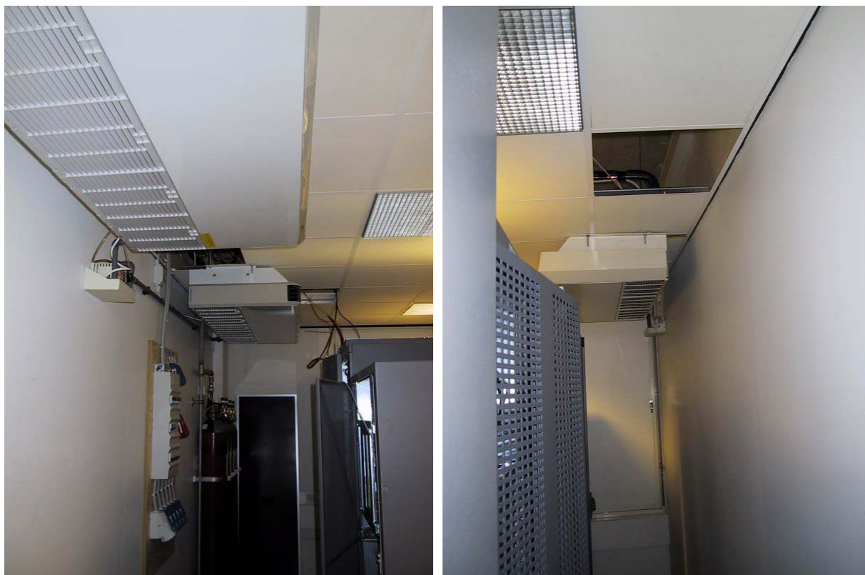
Figur 2. Serverrummets fordampere.
