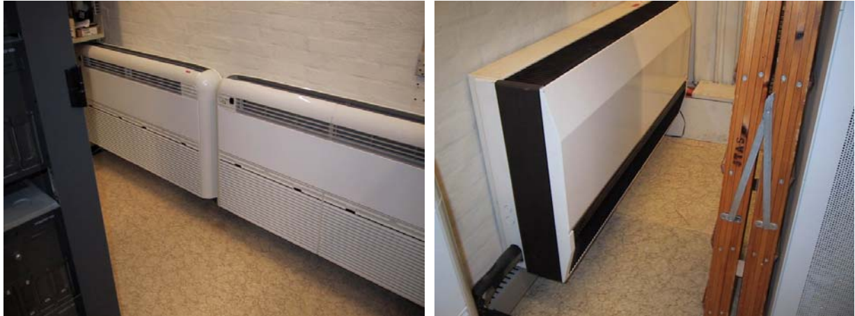
Figur 2. Serverrummets fordampere.
