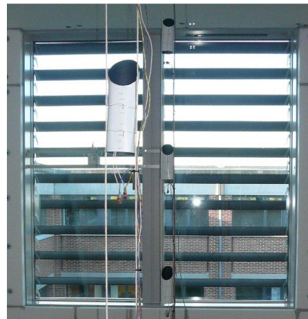
Figure 2 The view out of a traditional low-e window with solar control coating and external Venetian blinds in test room B.
