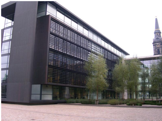
Figure 22 One south façade of the building.
