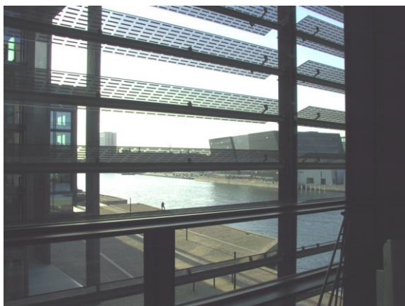
Figure 23 The external solar shading consisting of glass lamellas with silk screen printing.
